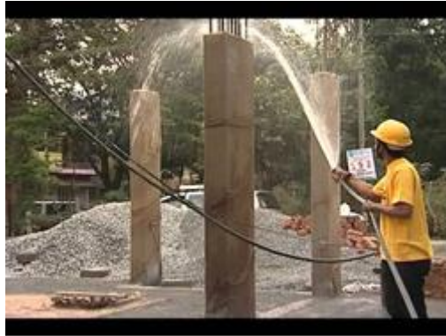
Gambar 8. Proses Curing
